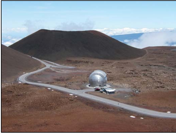
The CSO stands beside the Mauna Kea Access Road. Source: CSO
