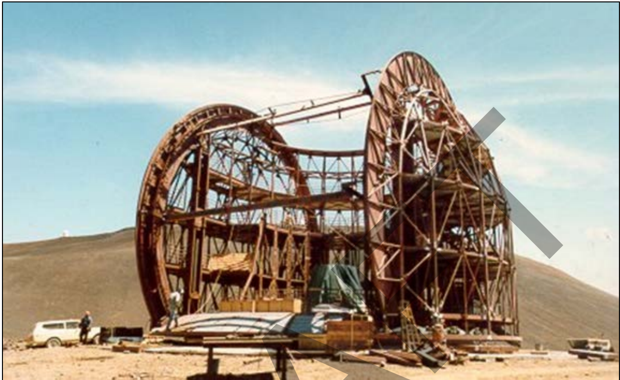
Figure 5-5: CSO's Internal Structure During Construction
